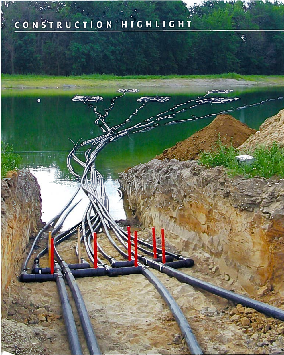
One third of the geothermal system's piping coils are in the pond. Attaching weights and filling the coils with fluid keeps this aquatic geothermal system submerged and in place.
