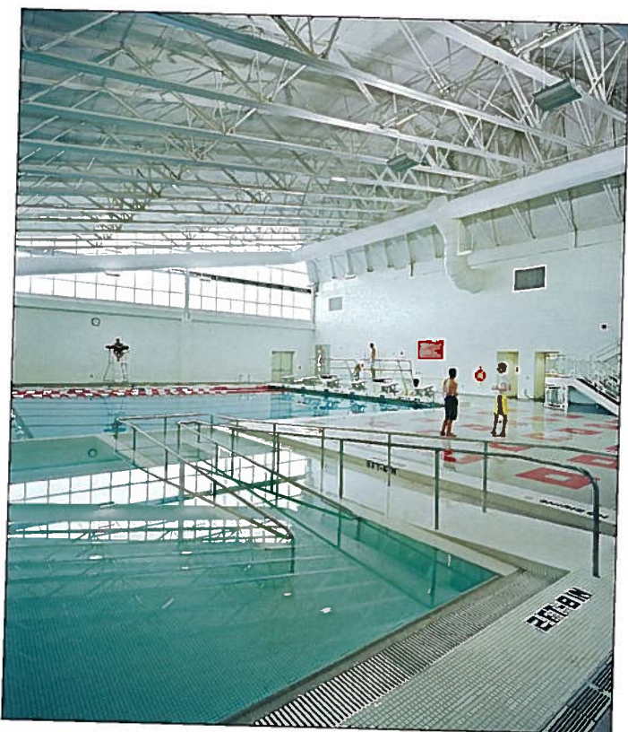
With air pretreated by a dedicated energy recovery unit, the community pool is yet another energy-efficient space in this 155,000-square-foot high school.
